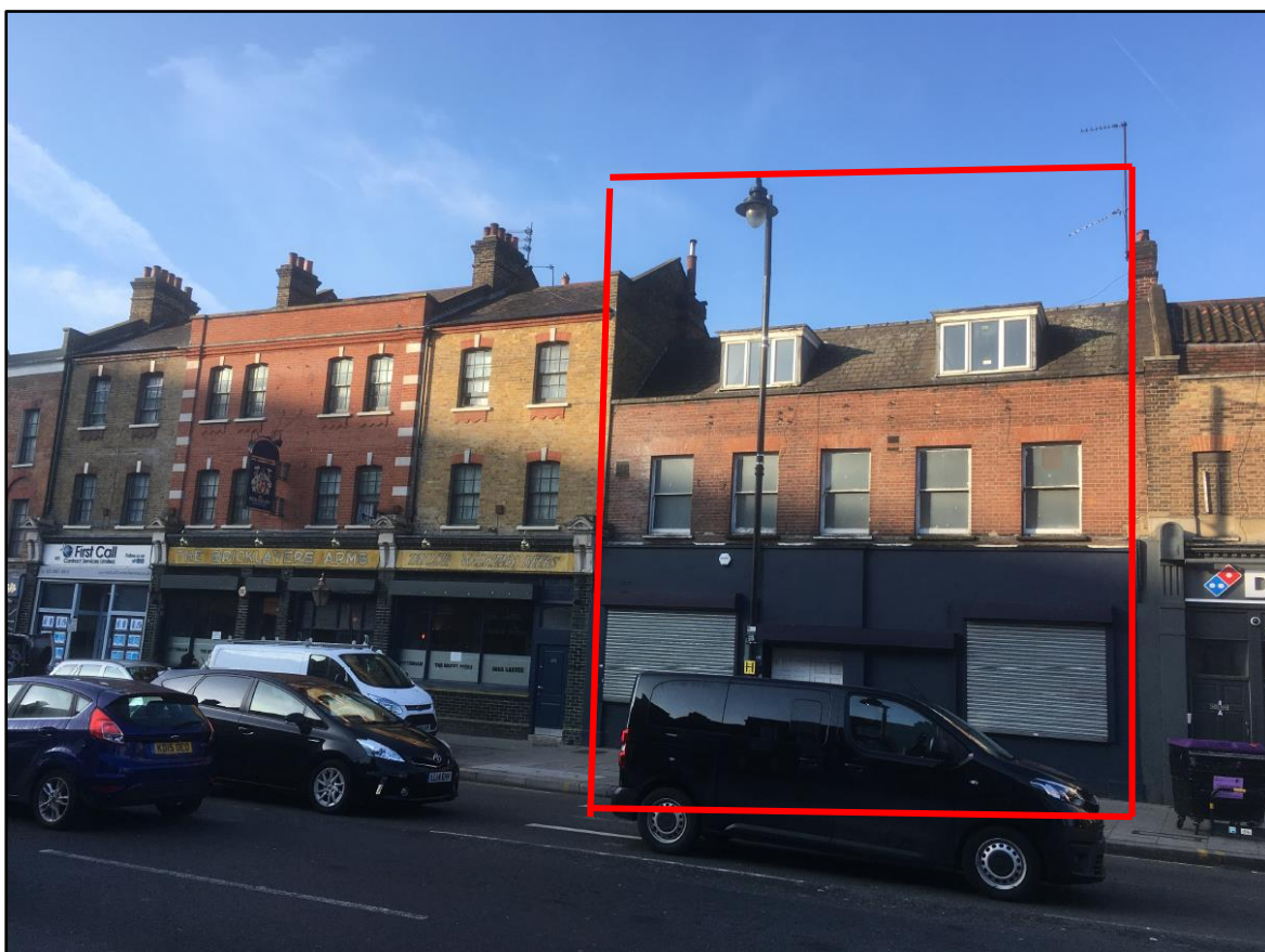
Existing High Road frontage
